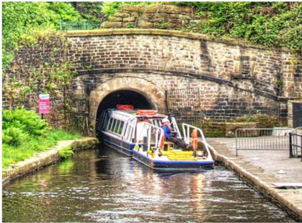
Entrance to Standedge Tunnel, Marsden, West Yorkshire, England. © 2008 54north Source: Wikimedia commons
