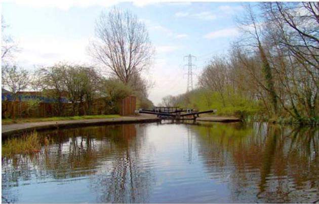
Upper pound, Lock 58 Rochdale Canal
