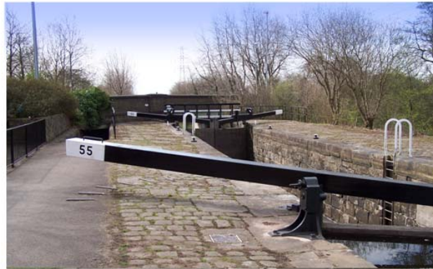
Lock 55 Rochdale Canal
